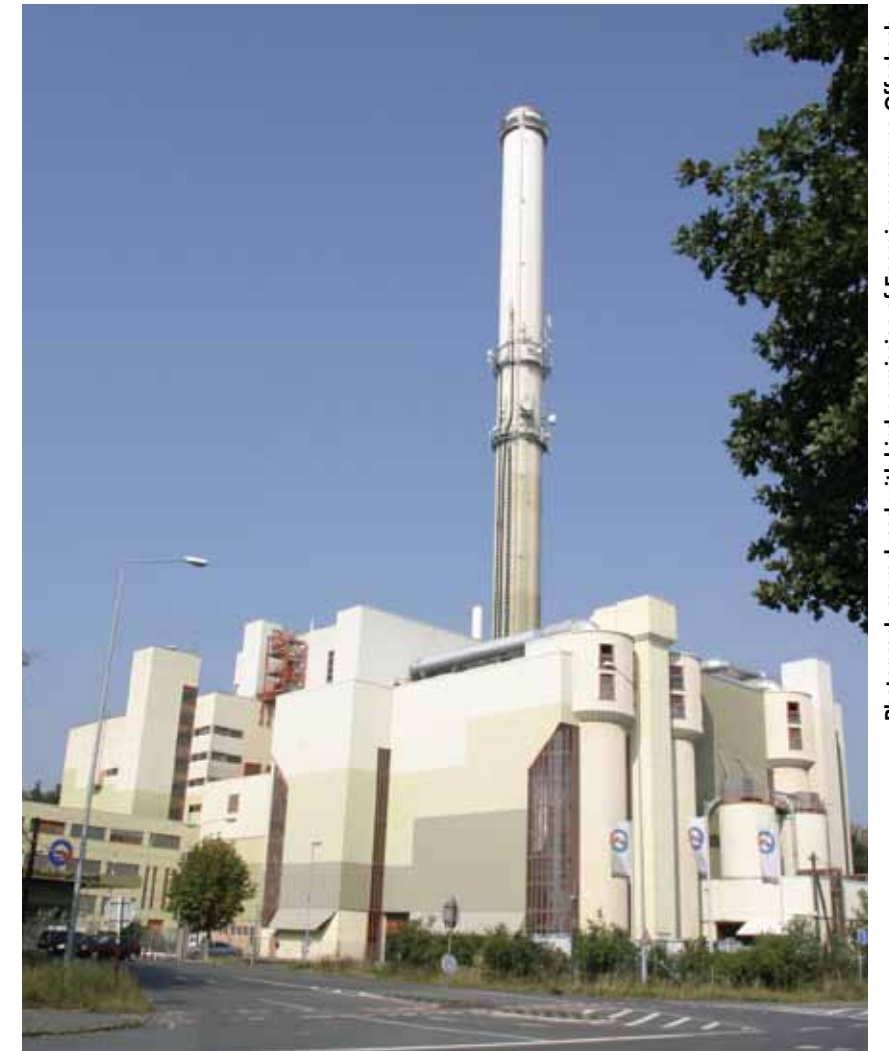
The MVV Offenbach plant in Germany, which processes 250,000 tonnes of waste
