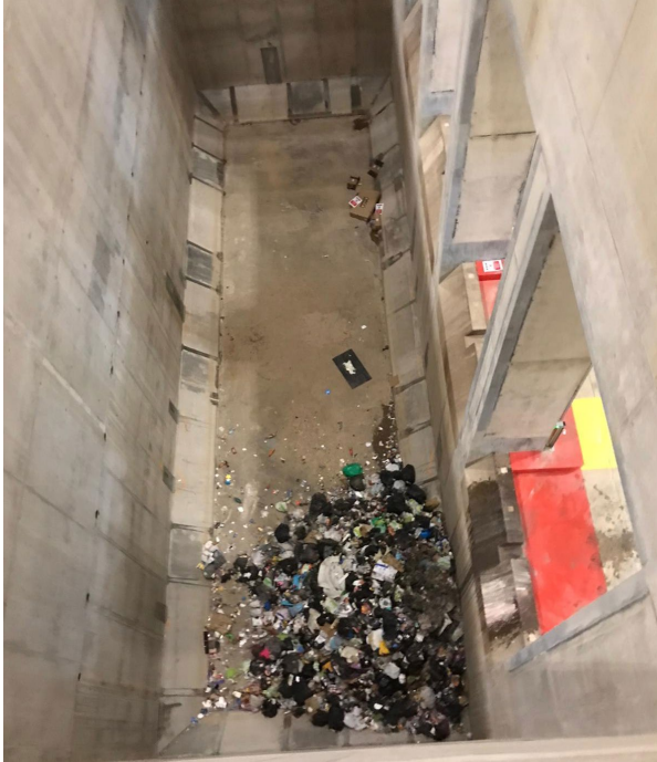
First waste delivered into the reception bunker in line 3
