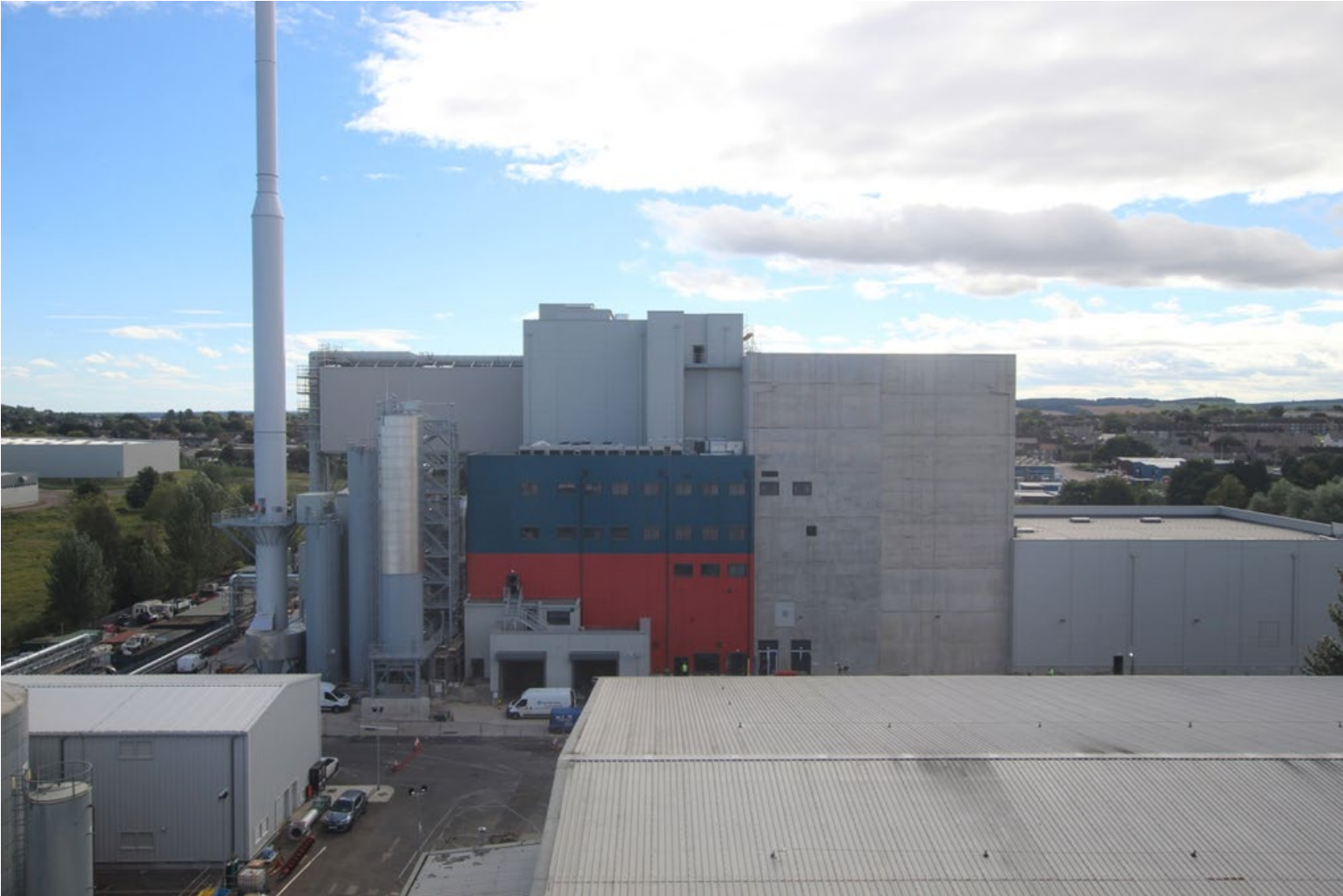
Actual construction site photo taken by Lobster Camera
