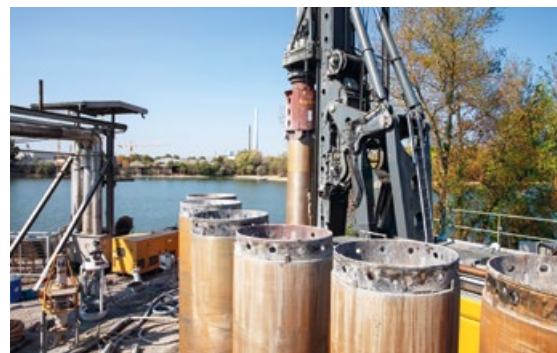
... and are progressing at full steam
