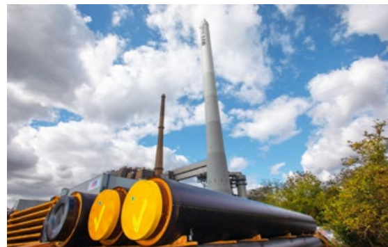
Preparations for the link are underway ...
