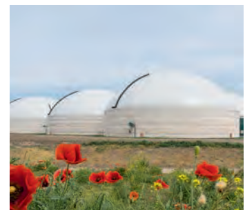
MVV Energie operates biomethane plants in the Magdeburger Börde region
