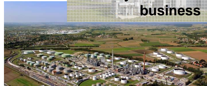
Joint district heating project in Ingolstadt
