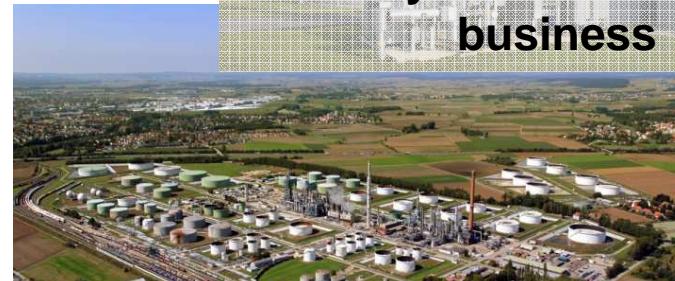
Joint district heating project in Ingolstadt
