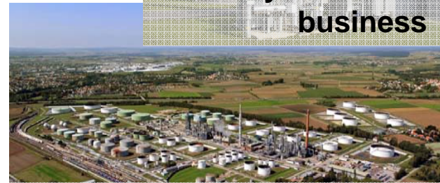
Joint district heating project in Ingolstadt
