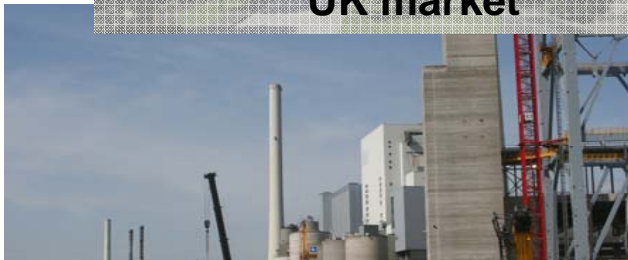
Expansion in district heating Block 9 GKM
