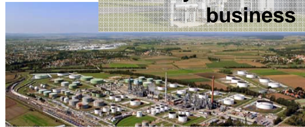
Joint district heating project in Ingolstadt
