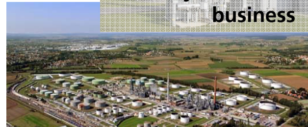
Joint district heating project in Ingolstadt
