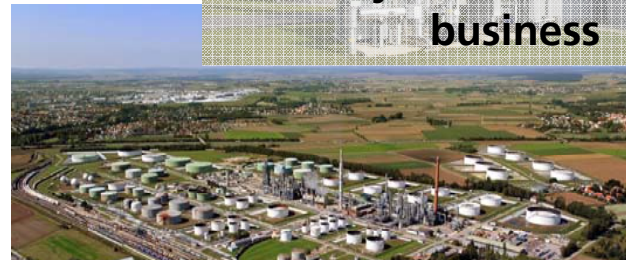
Joint district heating project in Ingolstadt
