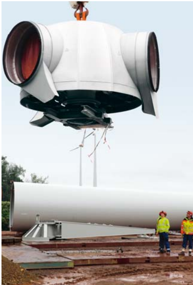
• Assembly work in Kirchberg – generating clean wind power
