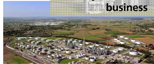
Joint district heating project in Ingolstadt
